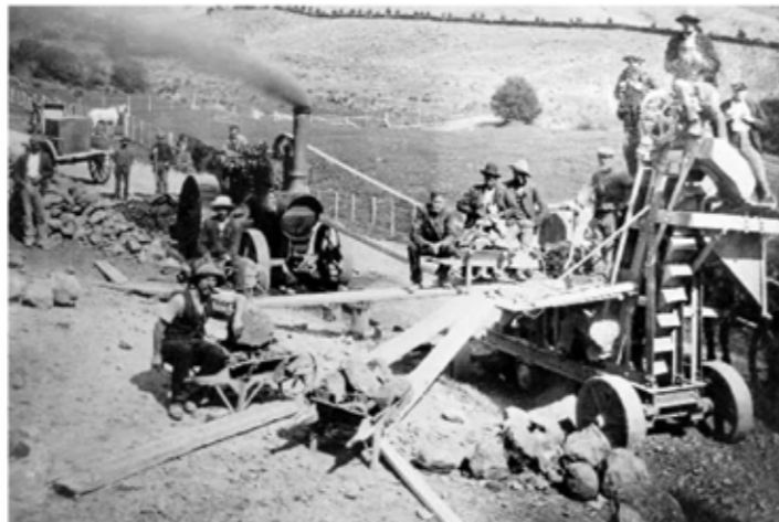
Photo 125: A steam engine used to drive a rock-crushing plant for road-making.
