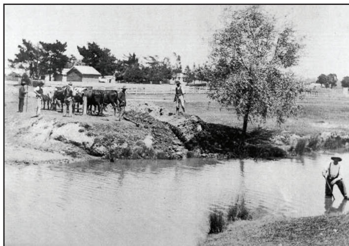
Photo 564: This picture comes from the collection of the late Gordon Cranny and probably shows the early stages of the construction of the first Woodend swimming pool on Five Mile creek. On the far side, a group of men are standing with a bullock team.
