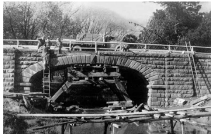
Photo 90: In 1958 the Woodend Bridge was widened by the Country Roads Board.
